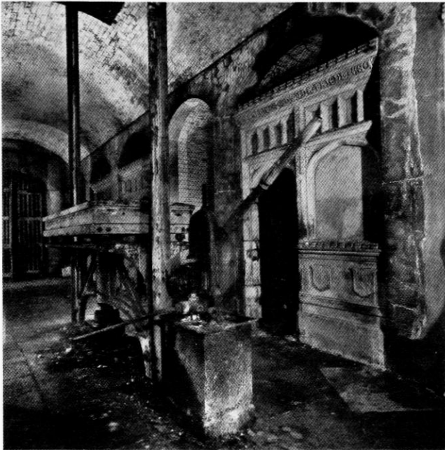
Hydraulic coffin lift or 'catafalque'. Photo by Nick Catford
